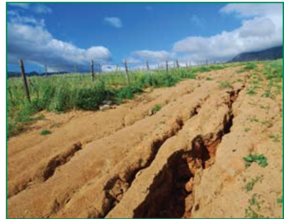
Typical erosion problem
